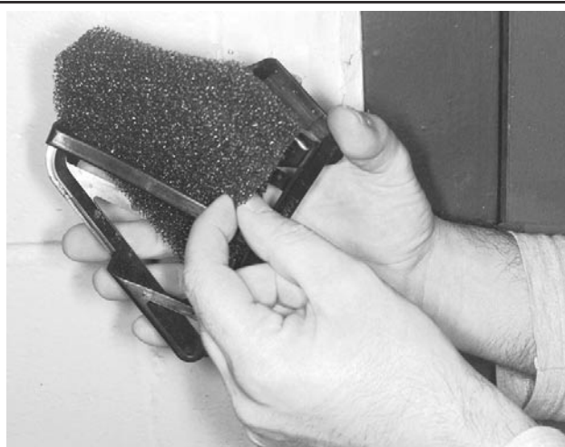
REMOVAL OF FILTER FROM ITS GRILL
