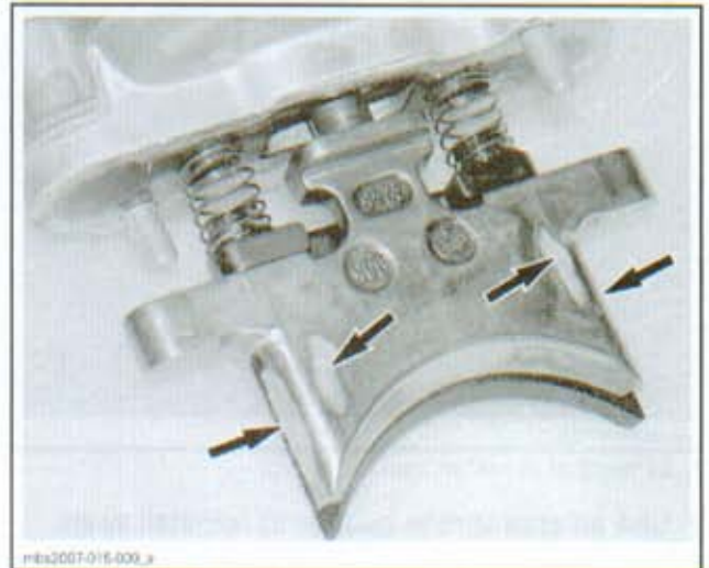
SIGNS OF WEAR
