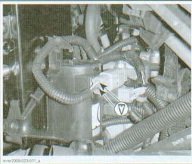
VOLTAGE MEASUREMENT AT CAPACITOR CONNECTOR
