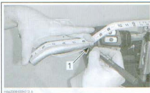
TYPICAL - MEASURING FOR HEATER POSITION
