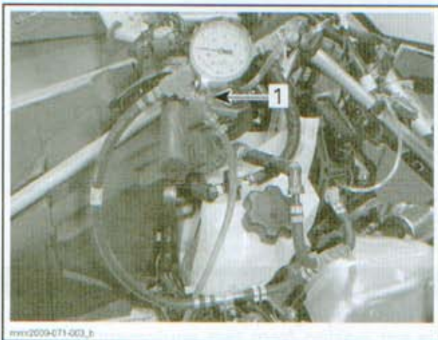
1. Pressure gauge bleed valve
